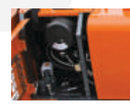
Ground level service access
