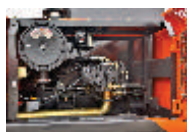
Ground level service access
